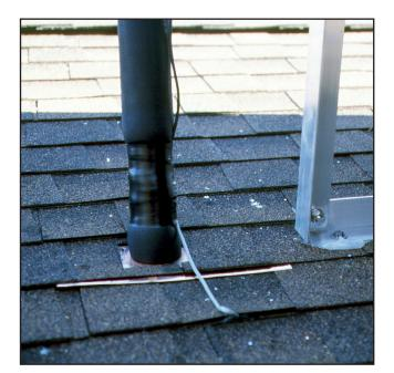
Completed installation of roof flashing with pipe insulation.
