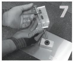
Slide the washer and the L-foot (not included) onto the lag screw.
