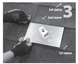
Insert flashing between 1st and 2nd course. Slide up so top edge of flashing is at least 3/4" higher than the drip edge of the 3rd course and lower flashing edge is above the drip edge of 1st course. Mark center for drilling.
