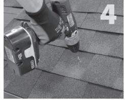
Using drill with 7/32" bit, drill pilot hole into roof and rafter, taking care to drill square to the roof. Do not use mount as a drill guide. Drill should be 'long style bit', aka 'aircraft extension bit' to drill a  $1\frac{3}{4}$ " deep hole into rafter.
