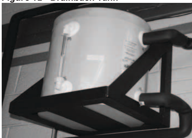
Figure 14 - Drainback Tank Relief Valve Piping
