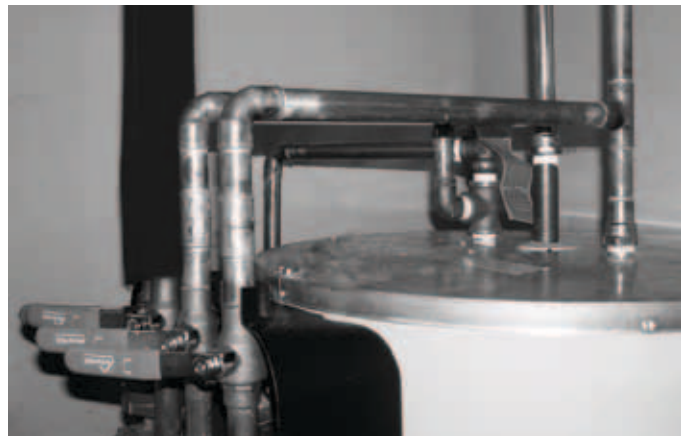
Figure 15 - SolVelox Piping
