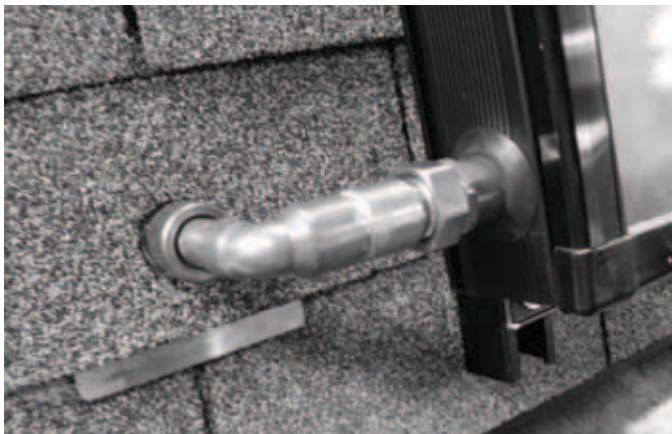
Figure 10 - Copper Flashing
