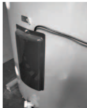
Figure 18 - Lower Tank Sensor
