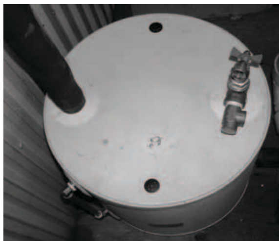
Figure 13 - Pressure Relief Valve
