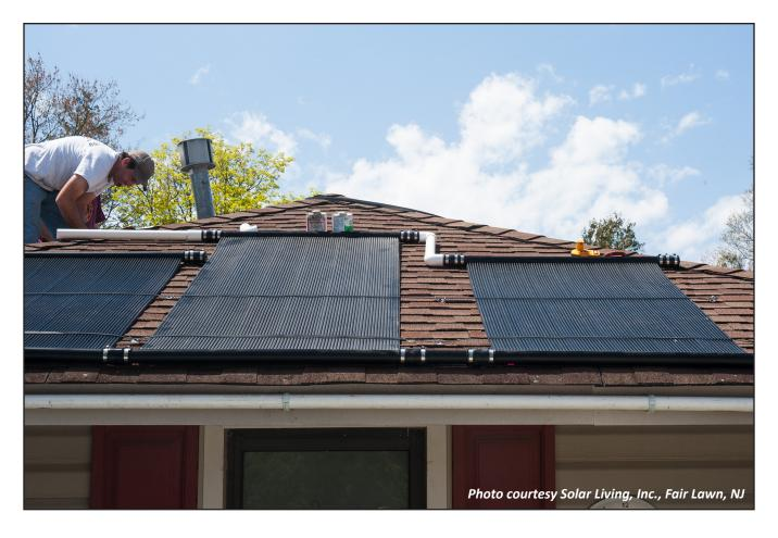
A typical situation that requires changing panel sizes. To maximize coverage on this hip roof, the panel sizes must be stepped up and back down.
