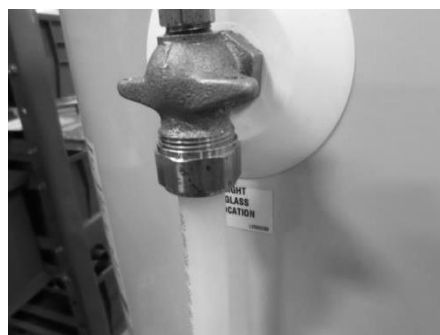
Figure 8 – Sight Glass Connected to Brass Fitting
