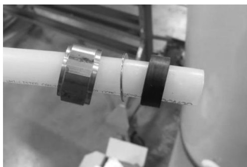
Figure 7 – Installing the Brass Fitting, Washer, and Gasket
