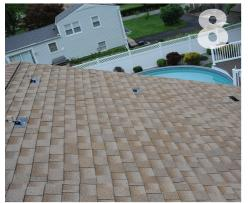
Install the low side strap mounts using the structural screws and the stainless steel/EPDM sealing washers only. Only install the bottom screw on the upper mount at this time, the upper bolt will be used later.
