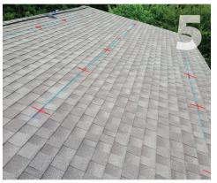
Lay out rough locations of all mounts using horizontal spacing specified in Aquatherm Installation Manual.
