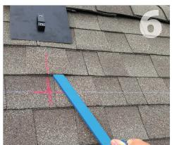
Remove any and all nails that will obstruct the Proper Flashing Placement (see pg 4). Use a roofing bar and take care not to damage the
