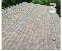
Snap chalk lines along the bottom of the strap mount flashings following the procedure from Step 1.
