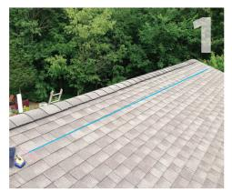
Lay out your system so the there is a small slope toward the inlet. Measure horizontal length of system and snap a chalk line across the roof at the location of the bottom of the header mount flashings.
