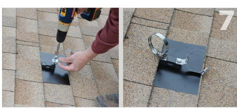
Install the first two header mounts using the EPDM gasket, the Aquatherm 50005 stainless steel bracket with stainless hose-clamp, the stainless steel/EPDM sealing washer and the structural screw. See page 1 for proper hardware sequence and orientation. Install 50005 brackets with hose-clamps on the bottom and the top of the mount. The bottom is for the header and the top is for the return line.
