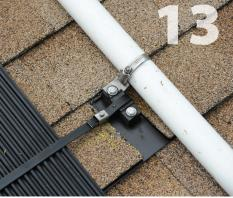
Use the top hole of the top strap mount on the low side of the system to attach a 50005 bracket with hose clamp. The bracket must be modified by removing a  $3/16^{\circ}$  x  $3/4^{\circ}$  notch out of the side. Solar pool heating system is now successfully mounted to the roof.
