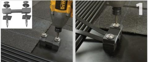
Install the flashed mount with the universal strap cap, leaving about a  $\frac{1}{3}$ " gap to allow for the installation of the strap. The  $\frac{3}{4}$ " x 1" EPDM gaskets go between the cap and the mounting block. The stainless steel/EPDM sealing washers go on top of the block as shown in cutaway above. Thread (weave) the strap under the block and back around between the block and cap. Pull the strap tight and finish tightening the screw.
