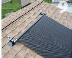
Install the first pool heating panel per the Aquatherm Installation Manual.
