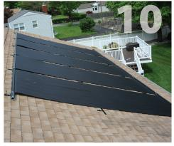
Install the next set of strap mounts and header mount and then install the next panel. Continue installing mounts and panels moving across the roof. Fine tune the locations of the mounts as each subsequent panel is installed.
