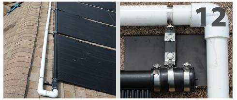
Refer to Aquatherm Installation Manual for return installation instructions. Fasten the return to each header mount using the hose-clamps installed earlier.
