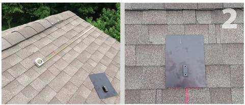
Lay out 1st header mount leaving enough room for access along the rake (edge of roof) or change in roof plane and with the bottom of the flashing at the butt edge of the shingle course. Choose a shingle course that will allow for the slope and still keep the top of the header mount flashing at the high side of your system below the ridge cap. Mark header mount placement.
