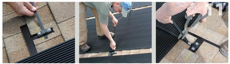
Install the strap by simply weaving it through the mounts and over the panels. When you get to the end, wrap the strap over the top of the mount and clamp it to itself, using the Aquatherm Strap Clamp, see pg 4 for use of the Universial Strap Cap. Cut off any excess strap. Be sure to keep the stainless steel clamp away from the panel.
