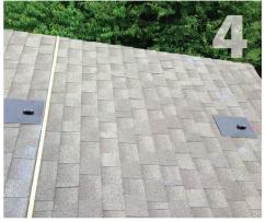
Lay out the strap mount locations of the low side of the system 4" from the 1st panel. This will allow room for clamping the strap without the stainless steel clamp rubbing on the panel.
