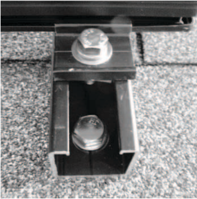
Figure 4b - Adjustable Mount Shown
