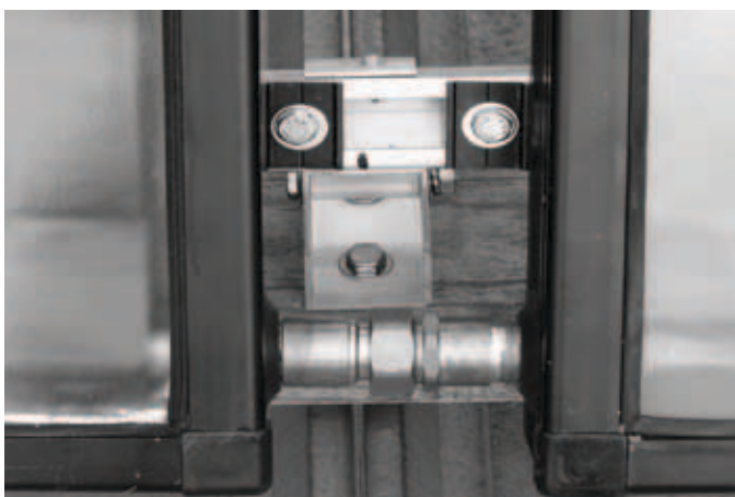
Figure 9: Joining Collectors
