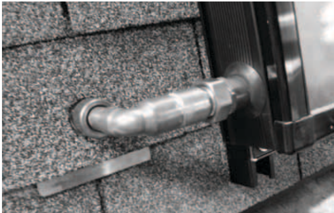
Figure 10 - Copper Flashing
