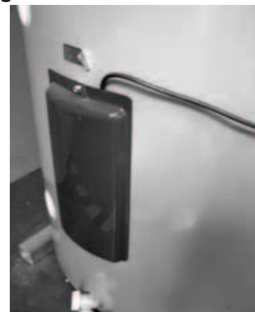
Figure 17 - Lower Tank Sensor
