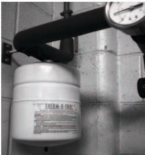
Figure 14 - Expansion Tank
