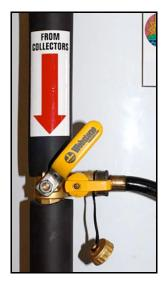
Step #1. This is the position of the Webstone combination purge valve handles for initial filling of the solar system. In this configuration the coil will fill first and automatically purge itself of air. After fluid runs smoothly proceed to step #2.
