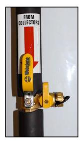
Step #3. This is the normal configuration of the Webstone combination purge valve for operation of the solar system. The ball valve is open, the drain valve is closed and the safety cap is in place to prevent accidental fluid loss. The valve must be initially installed in this configuration to operate properly.
