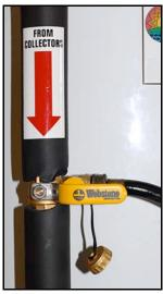
Step #2. This is the position of the Webstone combination purge valve handles for filling of the solar collector panels after the coil is filled. All air from the solar panels and piping will be forced out of the hose connected to the drain fitting back into the bucket used for filling the system. Once fluid starts flowing from the hose, gradually close the small drain valve until no more air is present in the fluid. After fully closing the drain valve proceed to step #3.
